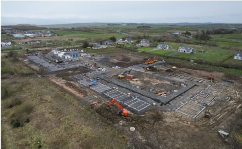
Image 1 - Progress photograph: Drumacrin , Bundoran
